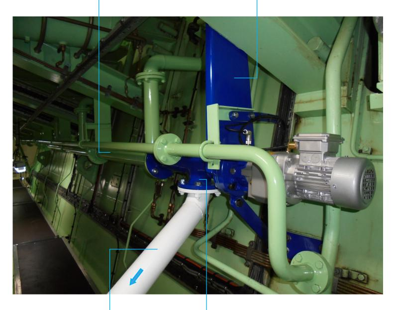
Sludge / oil outlet pipe leading to the sludge tank or <u>Sludge Collecting Unit (SCU)</u>  Tailormade adaptor pipe.
