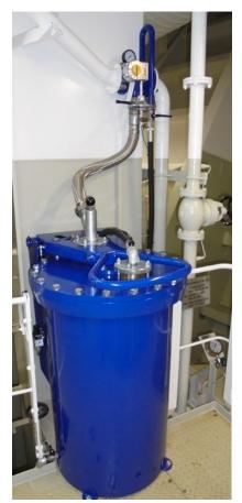
Sludge Collecting Unit (SCU) Effectively separates solid sludge directly into UN transport approved 210L standard steel drum.
