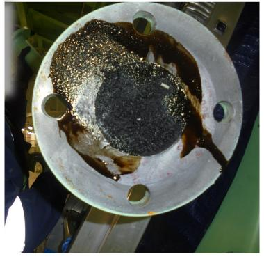
The partly or fully clogging of the drilled channel in the engine frame has a huge negative impact on engine operation:
